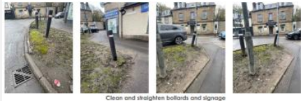
07 Material Clean & Replace
