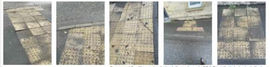
08 Pedestrian Crossing Material Replacement
