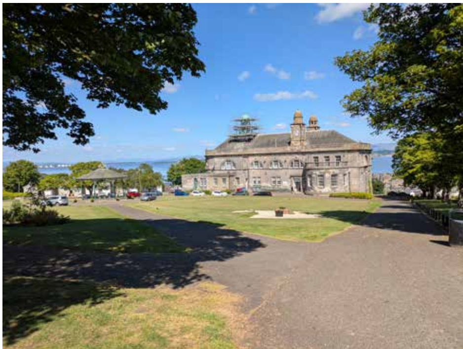
Site Image - Bo'ness Town Hall and Glebe Park
